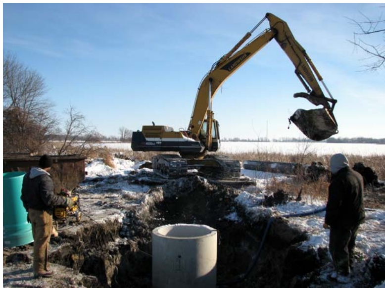
Installation of pipe on Smith Lake project
